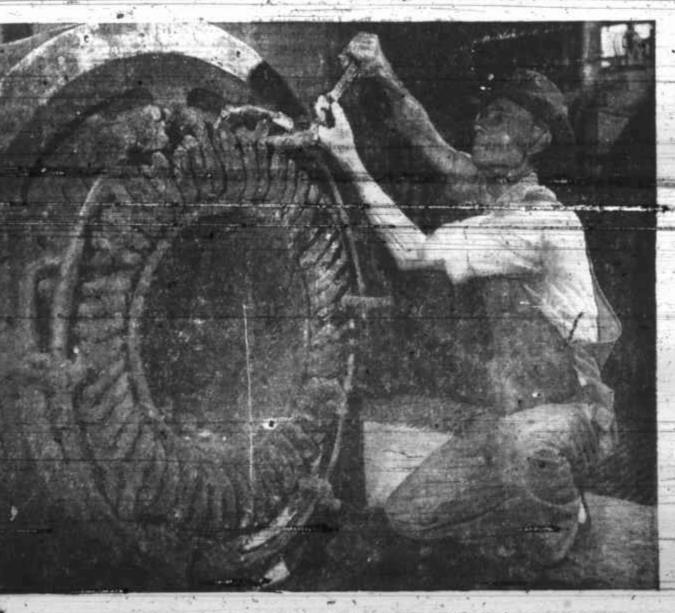
Partial view of 1500 kilowatt generator being dismantled by CPL Mechanic H. L. West,
